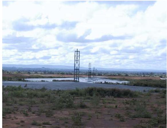
Photo 2: Early paste deposition – all towers viewed looking east (downgradient).
