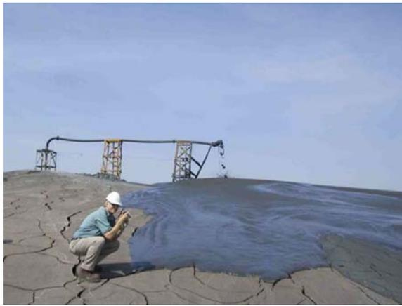
Photo 7: Advancing the tailings deposition with wooden trusses.
