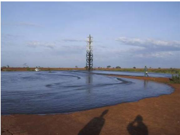
Photo 5: Early paste tailings flow at the start-up of the tailings basin. Note lack of free water.
