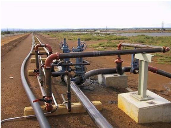
Photo 3: Valving along the main tailings line to direct paste and flushing water to individual deposition points.
