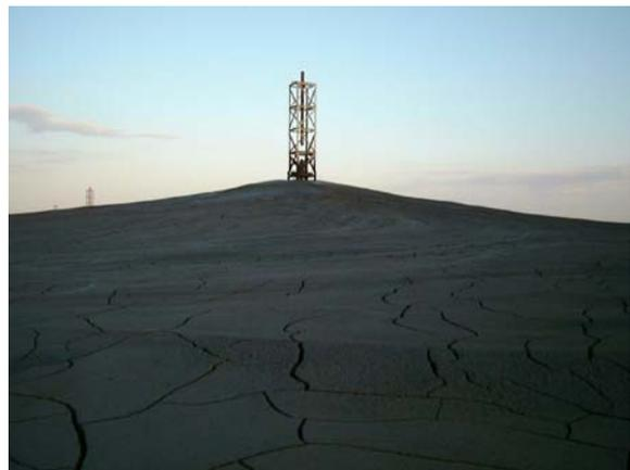
Photo 6: Progressive paste deposition forming a cone around a deposition tower.
