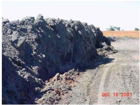
Photo 8: Excavation through desiccated tailings.
